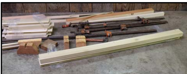
Figure 1: Precut door pieces and clamps for dry assembly.
